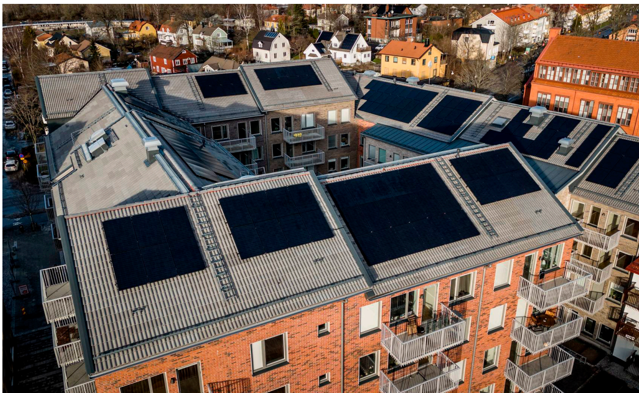
The extensive new construction and upgrade projects in Örebro in southern Stockholm include an entire block with energy-efficient buildings and climate-smart solutions. The surface of the roof has been utilised to install solar cells and the electricity they produce is expected to reduce John Mattson's purchased electricity by approximately 39,000 kWh/year.
